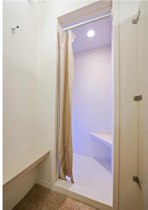
Newly renovated bathrooms at Yocum Hall, Univ. of Arkansas have solid surface surrounds, receptors and partitions, and feature a private, dry-floor changing space.
